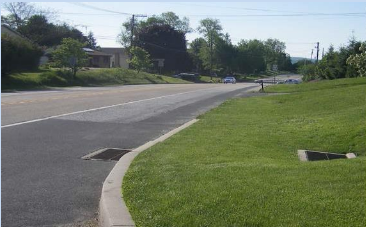
Figure 2.1.1- Conventional installation where enclosed surface storm water facility connects to highway storm water facility
