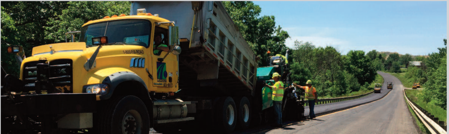
Recycled Asphalt Pavement being applied in District 1.
