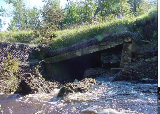
This top photograph shows settlement damage in the abutment due to scour taking away the earth underneath the abutment.
