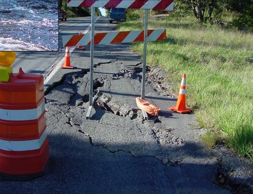
This is a photograph of extreme **settlement** damage in the abutment on the left-hand side of the photo.
