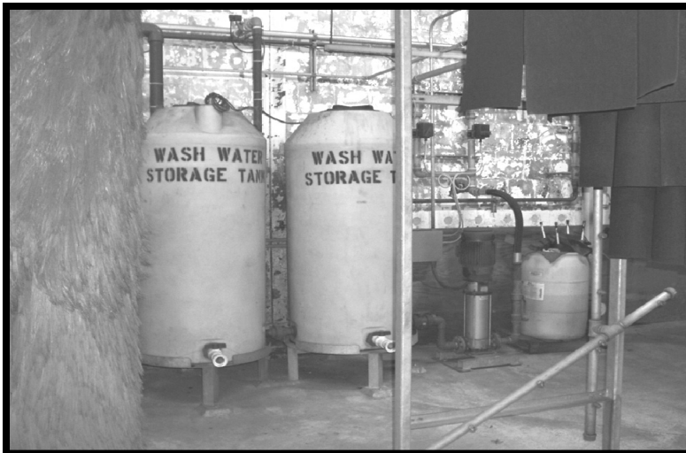
Storage Tanks for Recycled Wash Water
