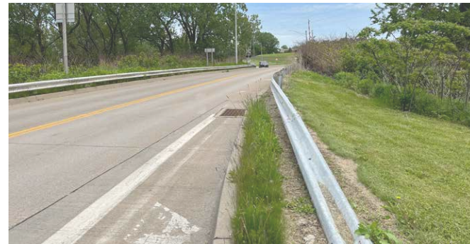
Pinchpoint with stormwater basin on the south side of Bay Drive
