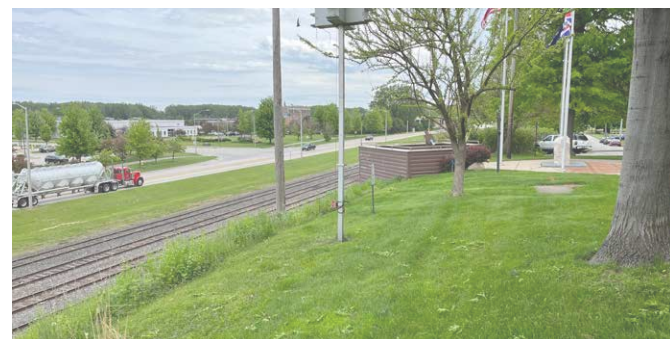
Steep slope and CSX railroad tracks north of Front Street
